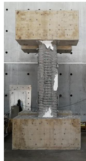
Figure 2: The column with the spiral reinforcement tested in MATS (Multi-Axial Testing System) at NCREE laboratory in Taiwan.
